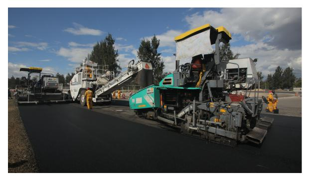
For this stage it is required over 50 workers and operators, besides supervisors. Once "Base Binder" is finished, the asphalt mixing plant will be calibrated again and placed at the complex Moises Solana to apply the last layer, the "Base Wearing" with 3cm thick.
