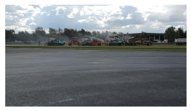
To carry out this process, three paving are used to avoid the longitudinal joint of fresh batch, and six steamrollers or compaction with tandem rollers, besides two transfer vehicles which are supplier machines that maintain the right temperature of the mixture and fill one by one. There is a fourth paving machine that will be used in Curve 1 which is one of the widest areas of the track with 19 meters. The asphalt mixture is used on the second and third layer, it is modified with polymers
